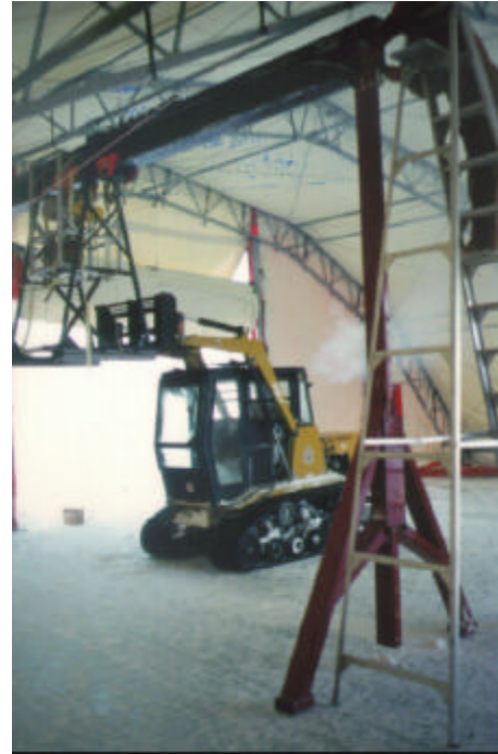
Figure 10. The I-beam is being bolted to its legs while the Posi-Track holds the I-beam in place.
